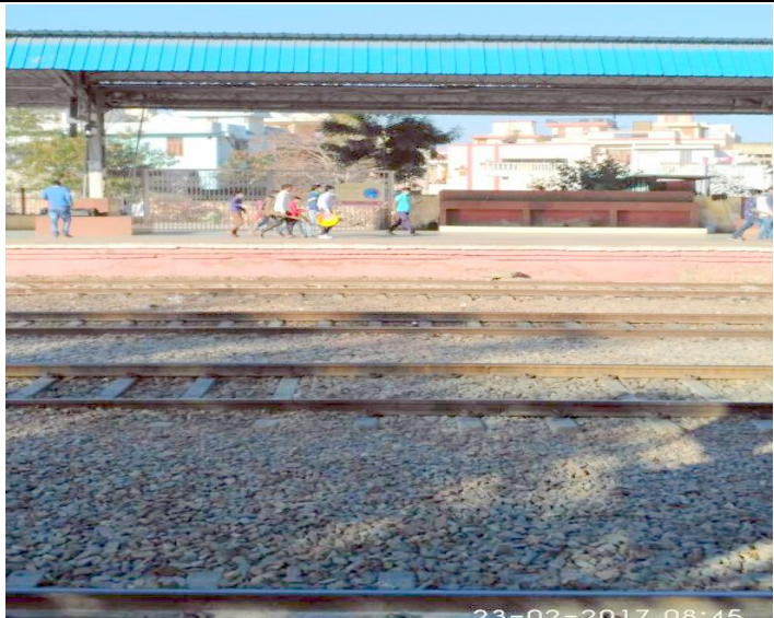
Cleaned track of GADJ station
